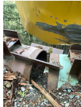
Pipe welded together
